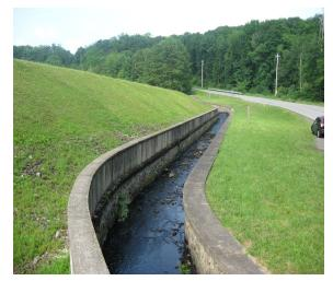
long earthen embankment dam. The crest of the earthen embankments is at El. 587.5. The embankment is approximately 20 feet tall at the maximum section.
